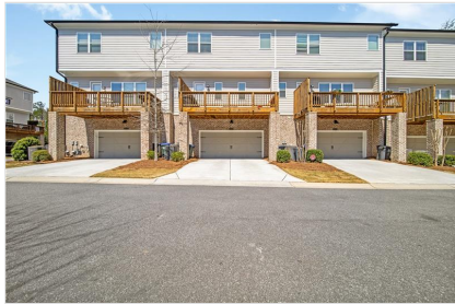
Front of Structure
