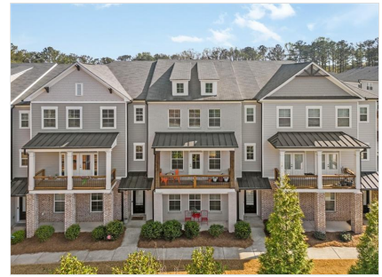
Front of Structure
