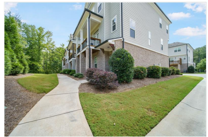
Side of Structure
